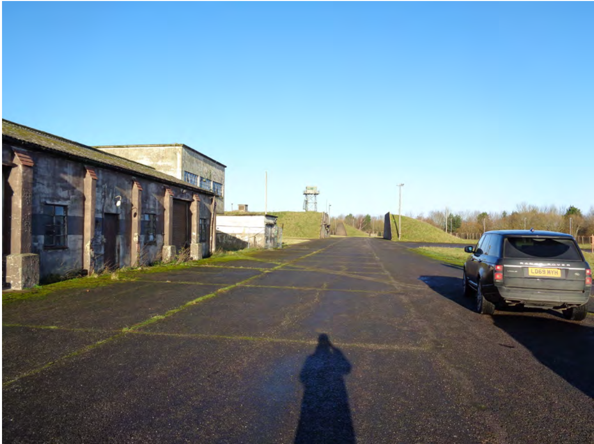
Plate 21: Buildings within the Scheduled Northern Bomb Stores, Upper Heyford airbase
