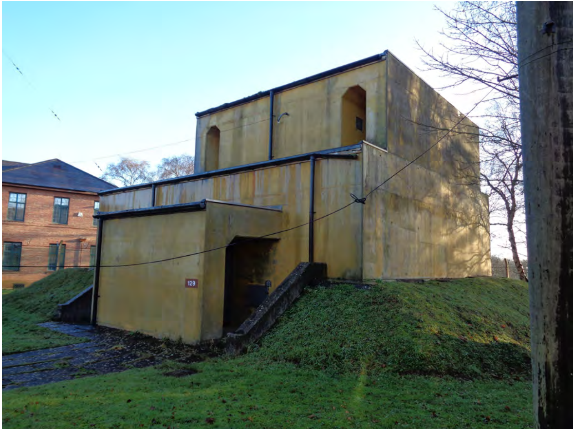
Plate 25: View of the Scheduled Telephone Exchange Building, within the Upper Heyford airbase
