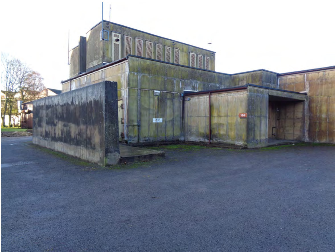
Plate 26: View of the Scheduled Battle Command Building, within the Upper Heyford airbase
